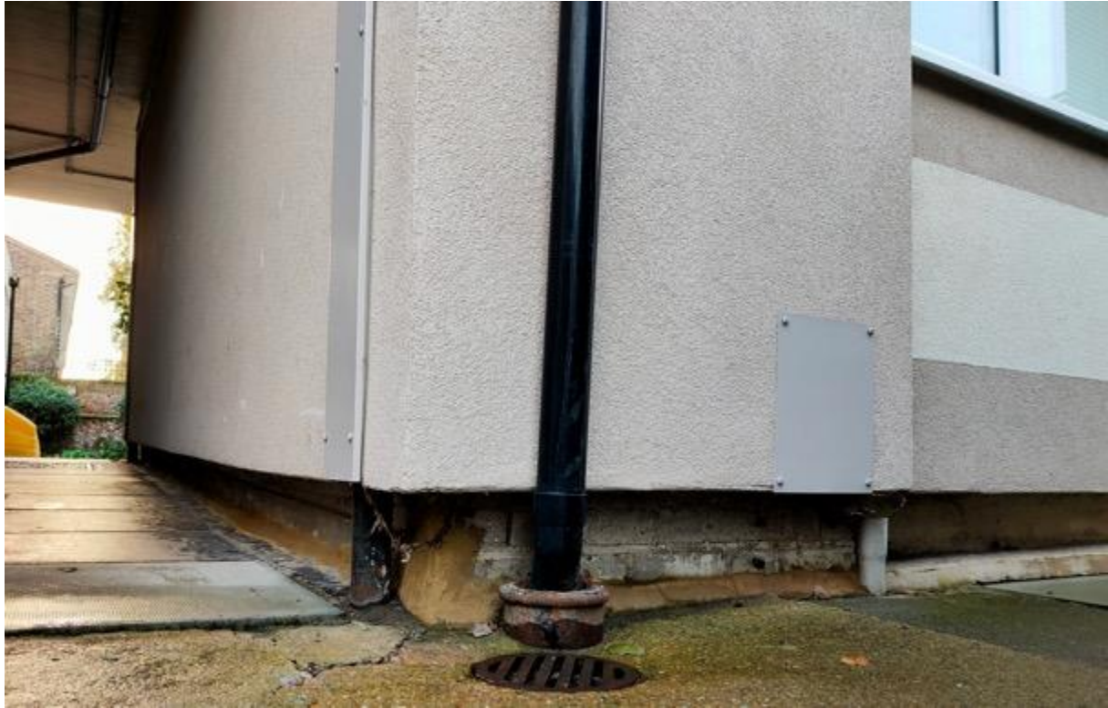
Looking outside one can see the cause of dampness. The mould lines up with the base of the wall where the retrofitted insulation starts. The gap is a normal, but it causes a thermal imbalance
