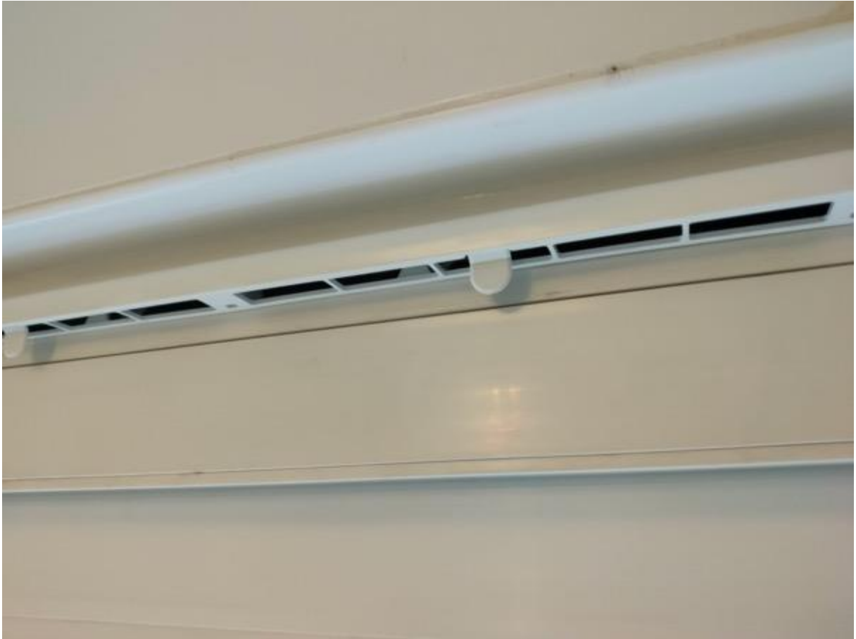
Trickle vents were closed. I opened them during the survey.
