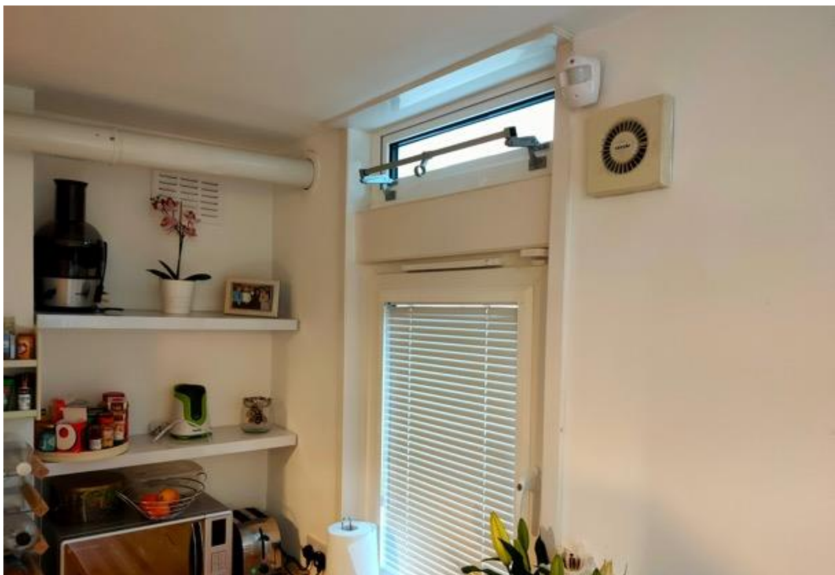
There is an extractor fan in the kitchen, but is it being use? Another solution is cook with tops on pots and pans and any indoor drying of clothes should be in a vented room with the door closed.
