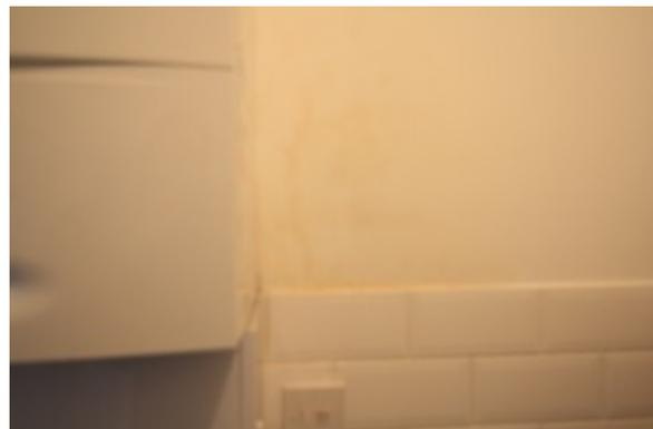
The image to the left shows extensive mould by the washing machine. The image to the right shows penetrating wall from a drip forming on the lower section of the upstairs' flat's boiler flue.
